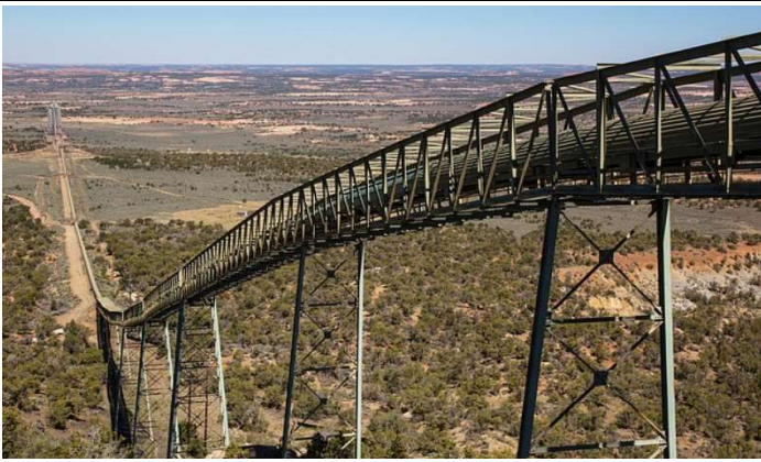
Kayenta Slurry Line
