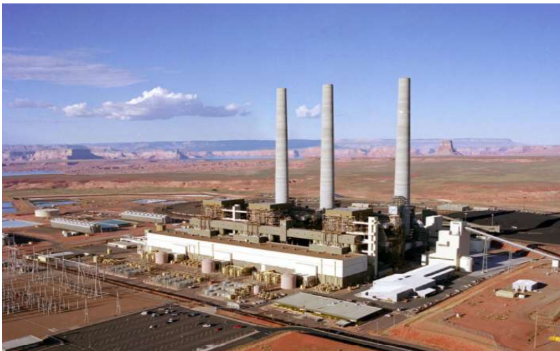
Navajo Generating Station
